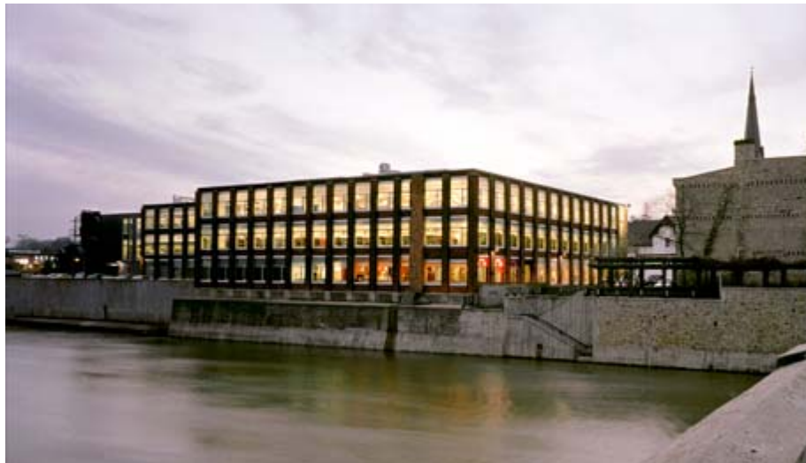
The University of Waterloo School of Architecture building in Cambridge, Ontario was insulated in part with rigid foam board insulation on the interior.
